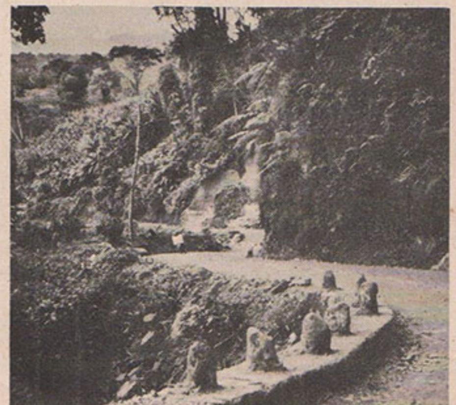
This is a typical section of the Pan-American highway as it enters Guatemala from Mexico. Carved from sheer rock in some areas, it travels from valleys to mountain peaks in just a few miles. Streams are often crossed on old wooden bridges, while beside them new concrete structures are still going up. Progress is slow here
