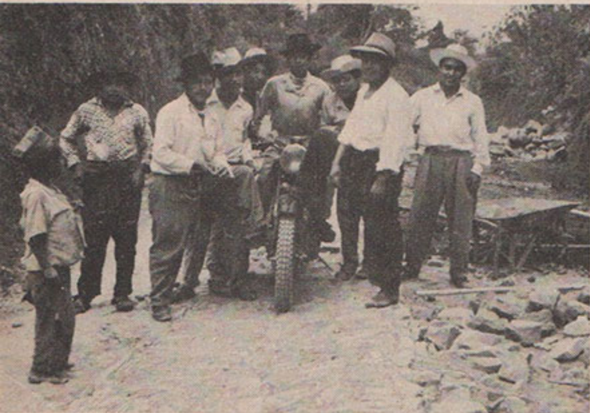
Life is just a bowl of "Cheeli Paapers" as far as these gauchos del camino are concerned. Ruta No. 1 was a mosaic masterpiece of small rocks placed on a bed of tamped earth. The spaces between were filled with more earth. I wanted a shot of this crew working, but the motorcycle and camera were too much for their curiosity
