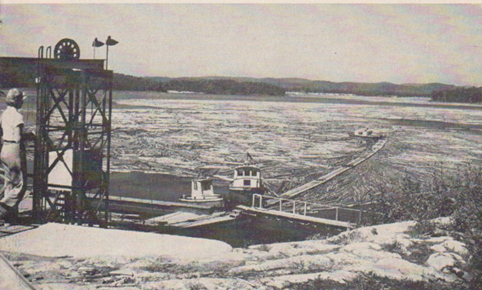
The pulp boom at Terrace Bay, Ontario. Ontario Dept. Travel & Publicity photo.
