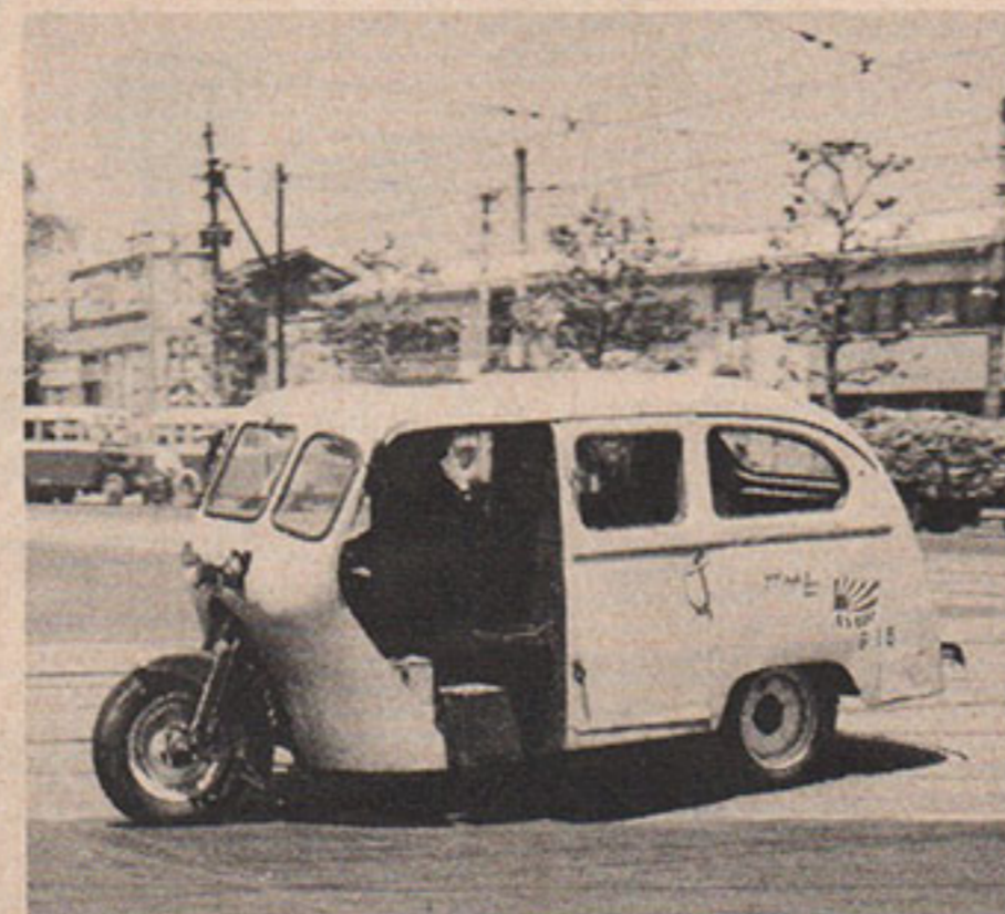
The Japanese have put motorcycles to more extensive use than have Americans. Three-wheelers fitted out with truck bodies or with passenger-carrying cabs are common sights on Japanese streets. This three-wheeler carries five passengers, three on automobile type main seat, two more on jump seat. Make of machine unknown
