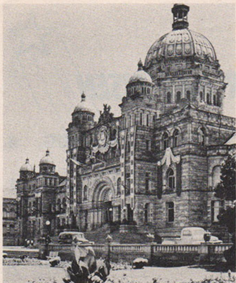
Parliament buildings in Victoria are festooned with banners and streamers in celebration of British Columbia's centennial year.
